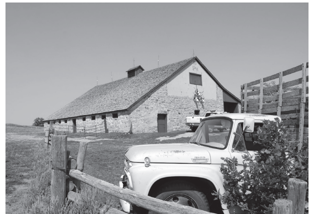
Anderson-Ridley Barn received a Deadwood Fund Grant to assist with repairing mortar and its walls.
